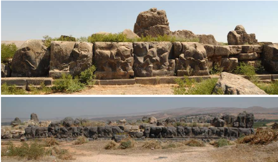
Fig. 3 Upper: Northwest facade. Lower: Southwest facade. Photos taken by T. Hayashi in 2007
